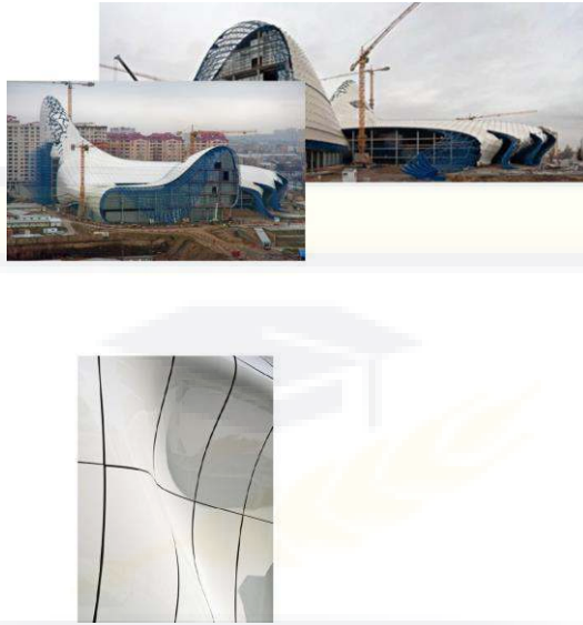
Gambar 4.12 Material Glass fiber reinforced plastic (GFRP) dan glass fiber reinforced concrete (GFRC)
