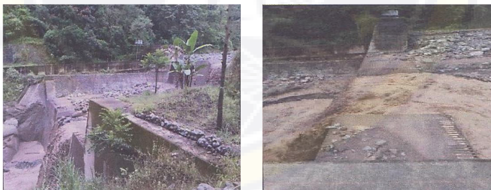
Gambar 3. Sabo Dam No. 7-1
