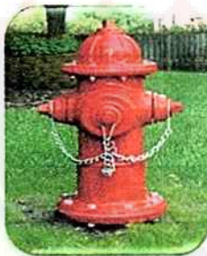
Gambar 5.26 : Water Hydrant (Sumber : www.google.com )
