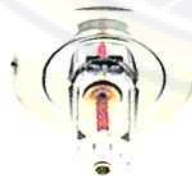
Gambar 3.19 : Water Sprinkle (Sumber : www.google.com )
