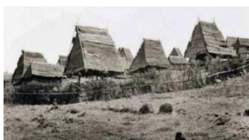
Figure 1. The Condition of Uma Lengge in 1993
