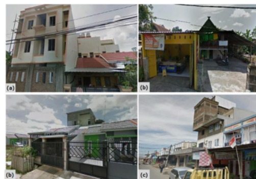
Figure 8. (a) converting and renovating a dwelling to a boarding house; (b) filling the space through the alteration of the yard of a type 21 house and the underbelly of a stilt house, (c) adding floors and roofs to a shophouse complex Source: Author's elaborator
