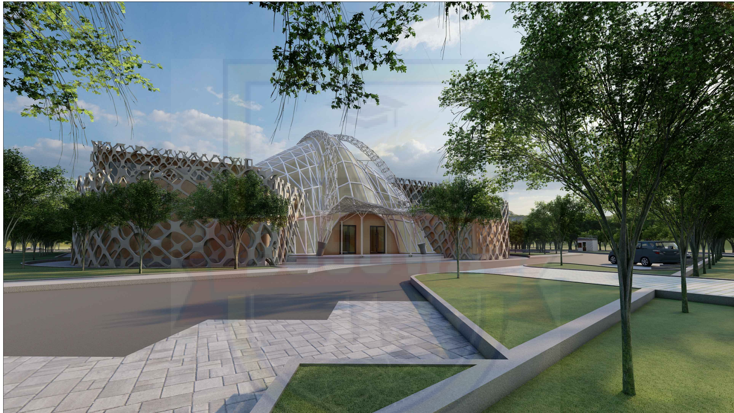
EXTERIOR VIEW BELAKANG
