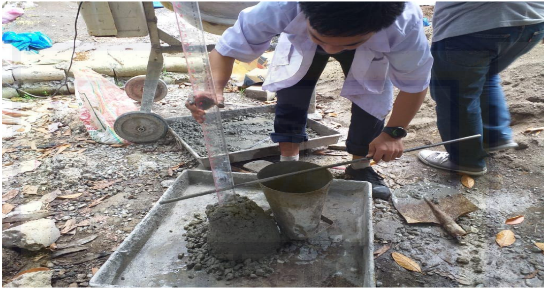
Proses Test Slamp Beton
