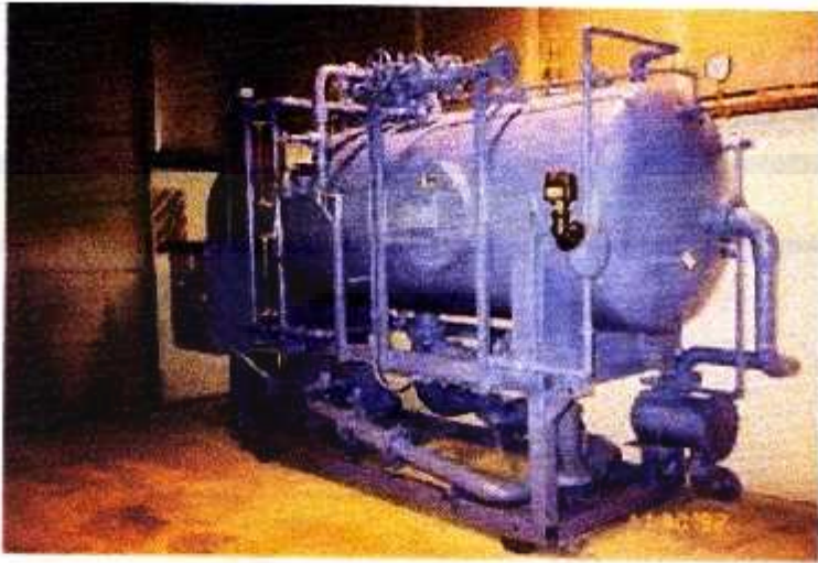
Gambar boiler pipa air
