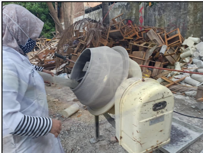
Gambar 4.22. Proses campuran beton
