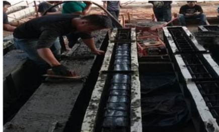
Figure 5. Casting of specimen.
