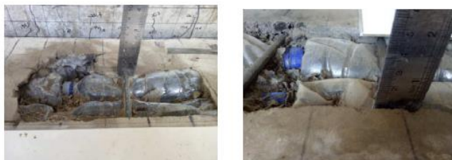
Figure 8: Measurement of concrete blanket thickness on HB2C 1 and HB2C 2 beams
