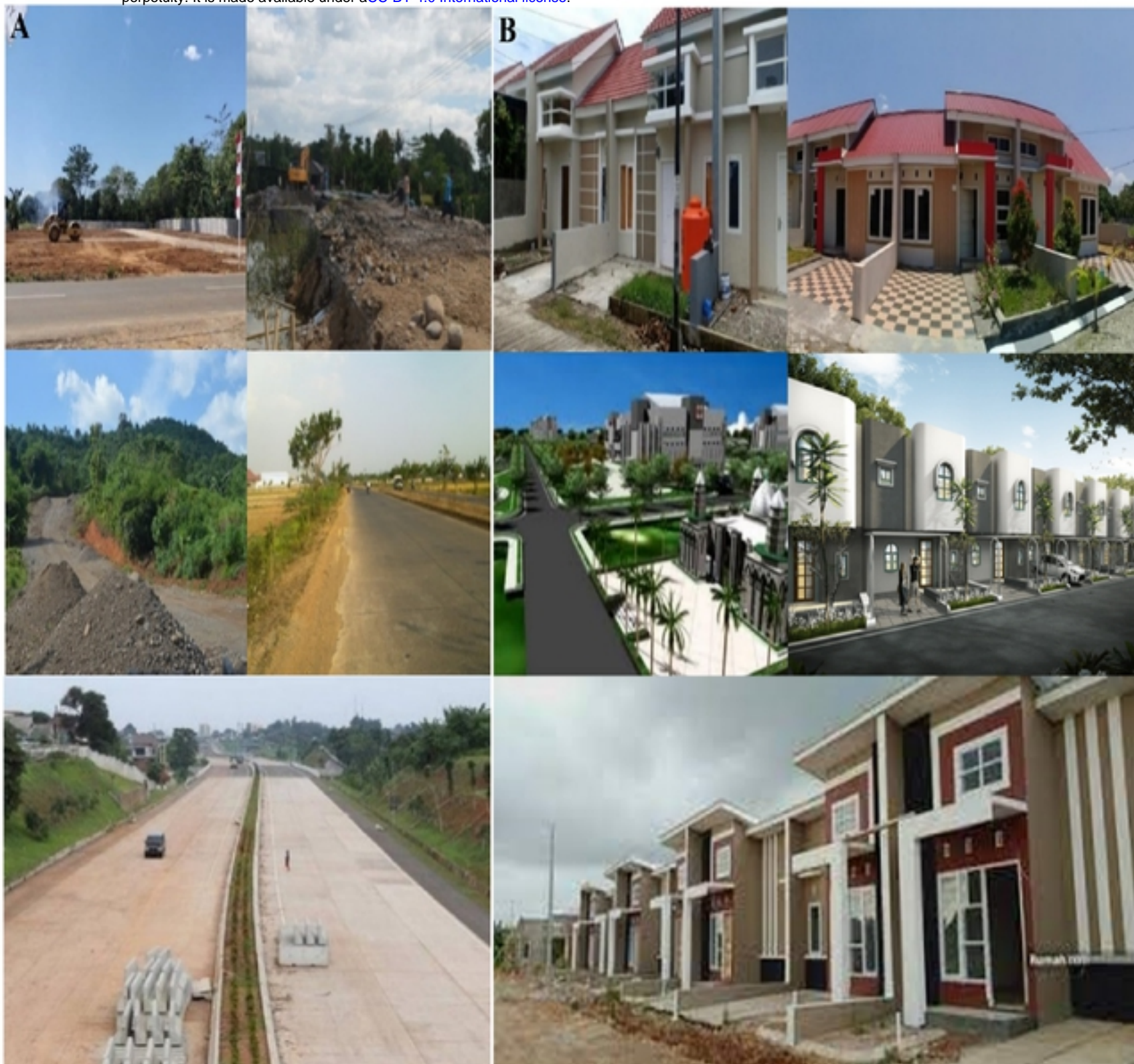
Fig. 2. (A–B). Development of the new city area of the Moncongloe-Pattalassang. (A) Land reclamation and road infrastructure development; (B) Housing development and socio-economic activities.
