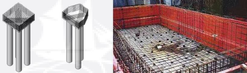
**Gambar 5.11** Pondasi *Bore Pile*
