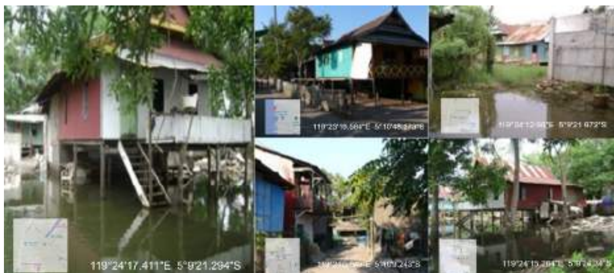
Figure 7. Slum Residence in new metropolitan areas of Metro Tanjung Bunga
