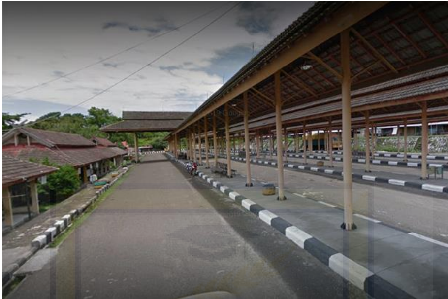
Gambar IV.8 Terminal bus Pare-pare
