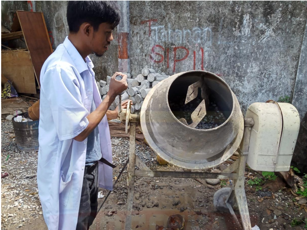
Proses Mix Material beton normal
