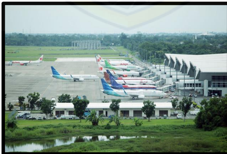
Gambar 4.7. Taxiway Bandara Sultan Hasanuddin
