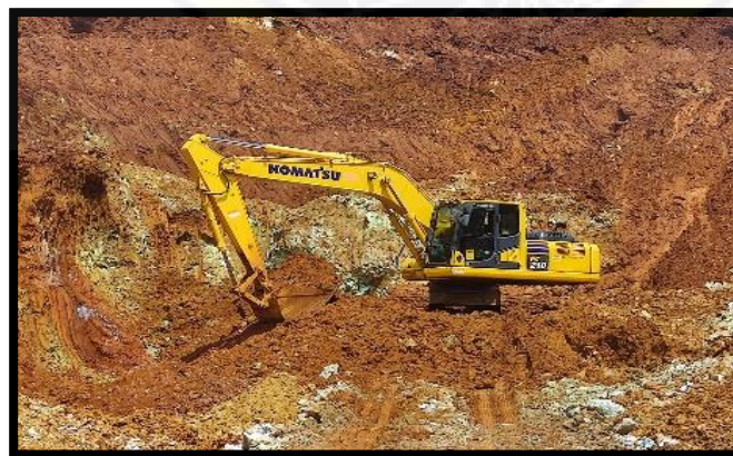
Gambar 2.3 Excavator Komatsu Pc 210 (Rifky hidayat 2022)
